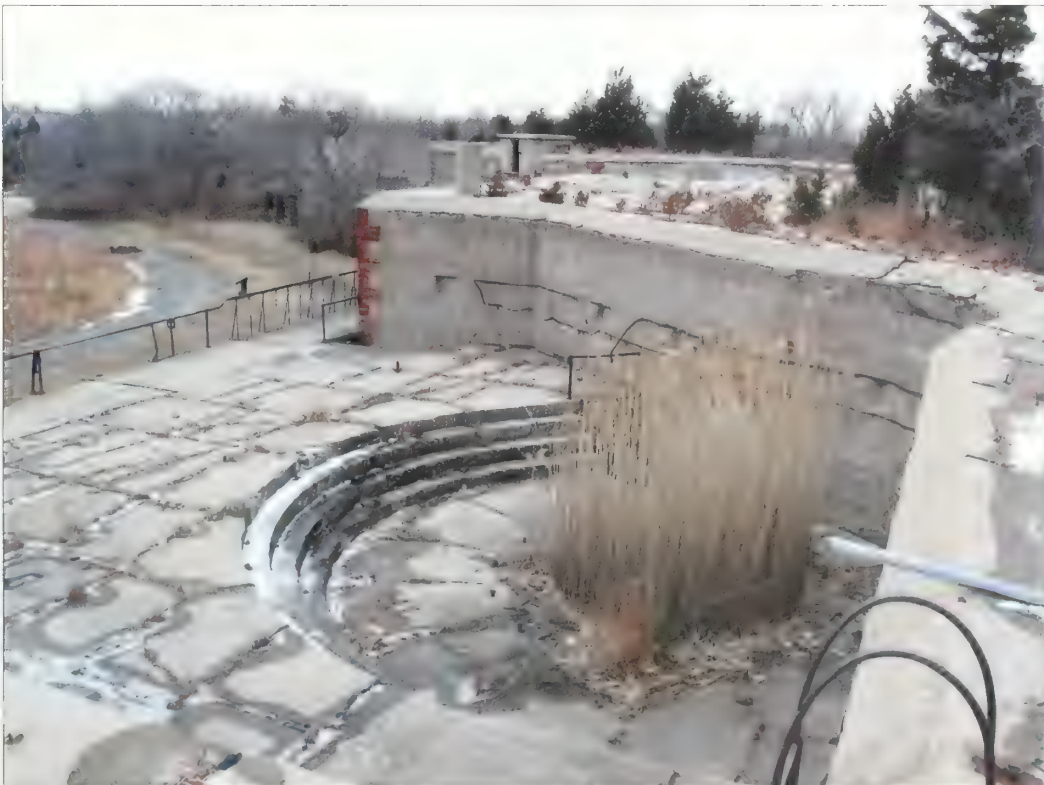
Figure 3.22. View looking west at emplacement #7, Nine Gun Battery. Phragmites ( Phragmites sp.), also called common reed, is growing in the gun wells at emplacements #6, #7, and #9 (Olmsted Center, January 2009).
